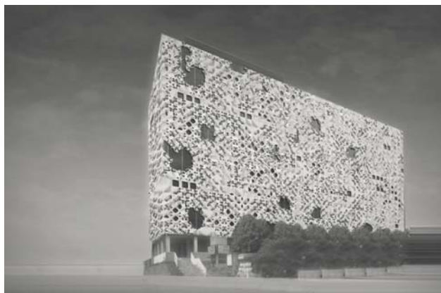
Kol/Mac architecture – INVERSAbrane - high-performance exterior building, membrane prototype, 2006. Source: Y. Grobman and E. Neuman, Eds., Performatism: Form and Performance in Digital Architecture . Routledge, 2011. P. 120-121
